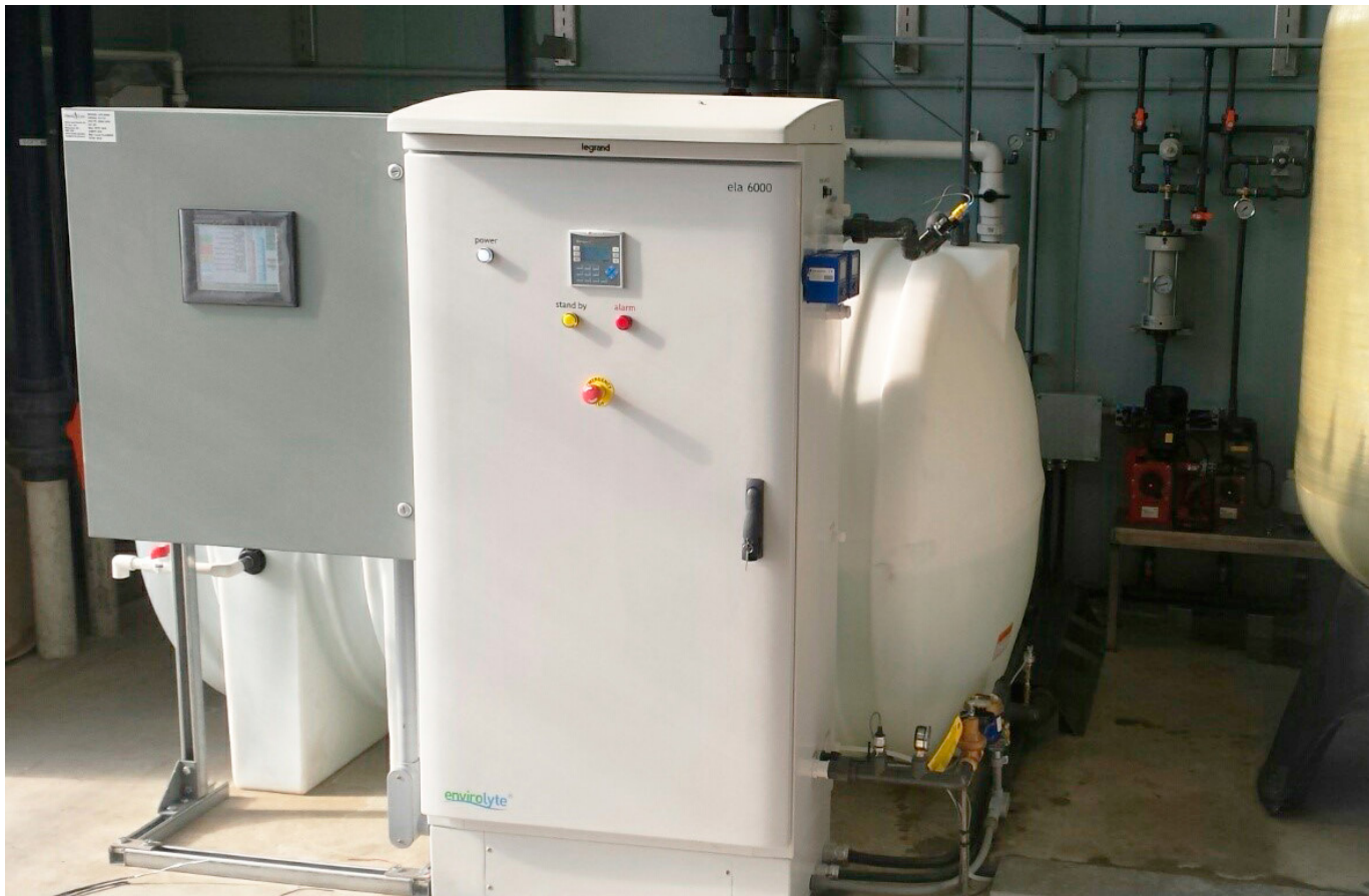
On site installations of ela6000
