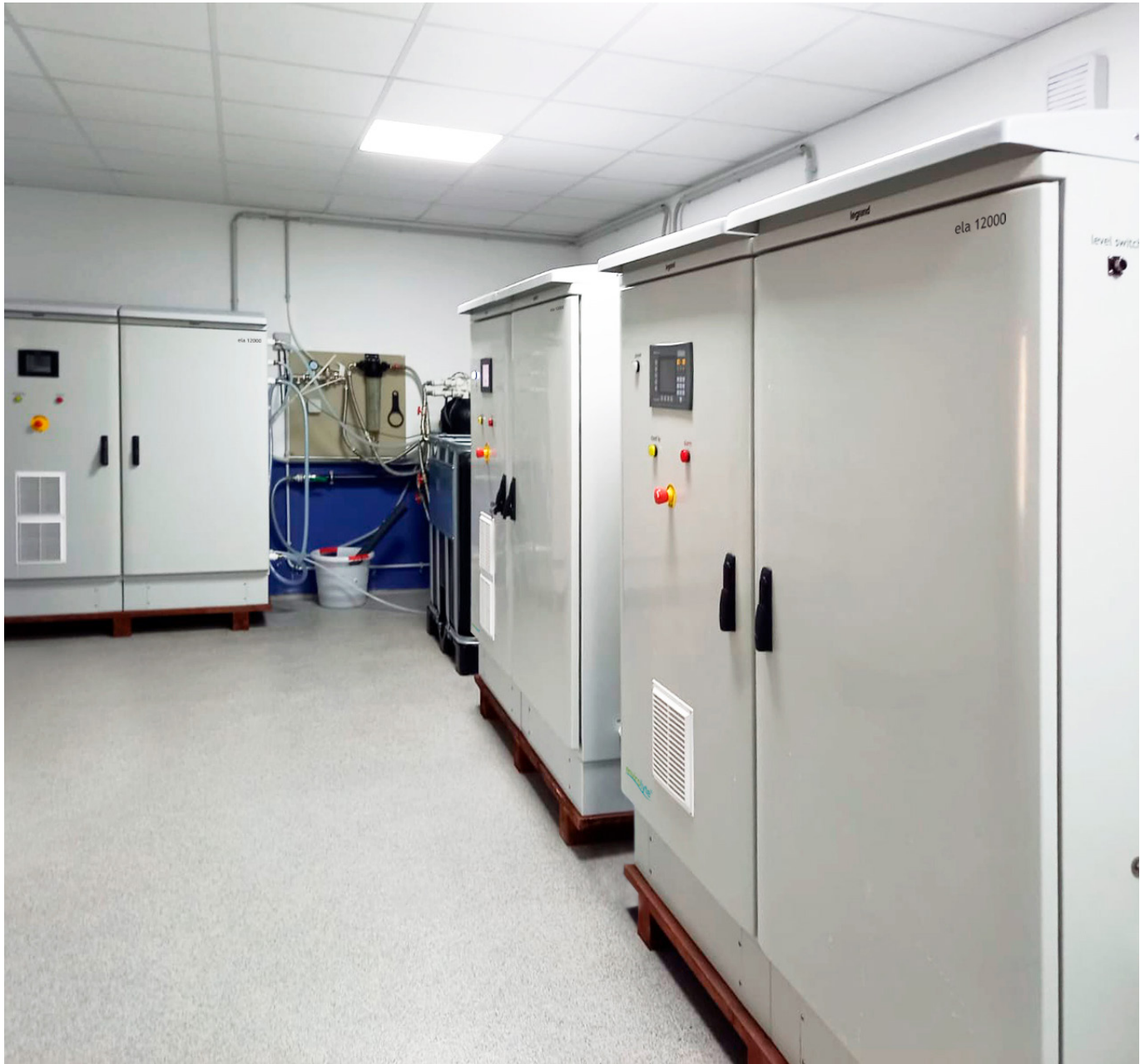
On site installations of ela12000
