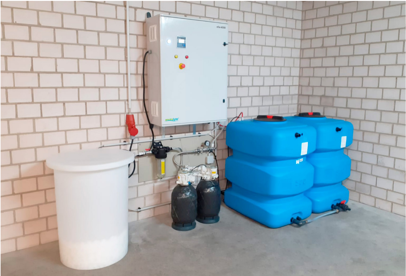
On site installations of ela4000
