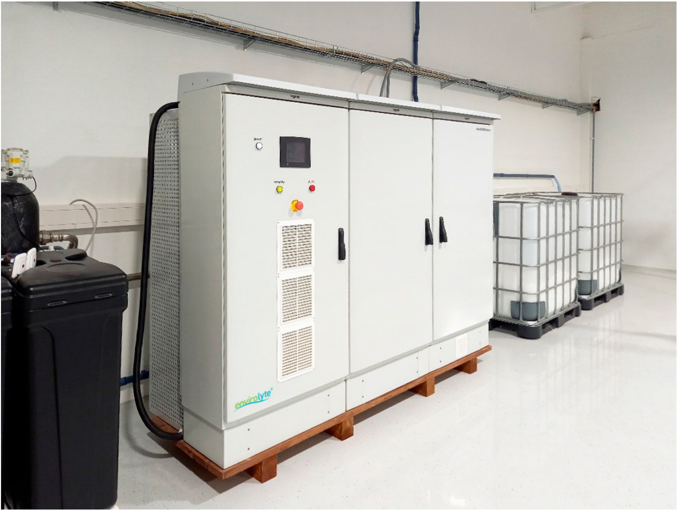
On site installations of ela60000ANW
