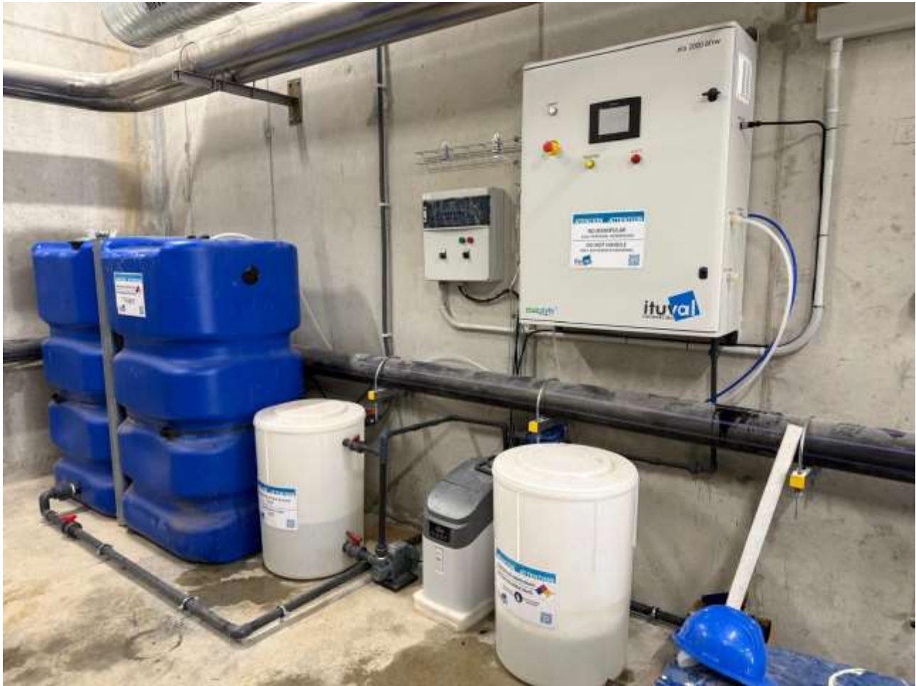
Envirolyte ELA - 2000ANW with brine tank, storage tank and water softener
