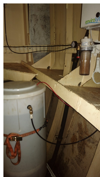
Different elements of the installation: anolyte tank, dosing pump and brine tank
