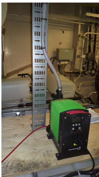
Different elements of the installation: anolyte tank, dosing pump and brine tank
