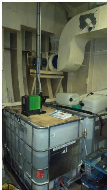
Different elements of the installation: anolyte tank, dosing pump and brine tank
