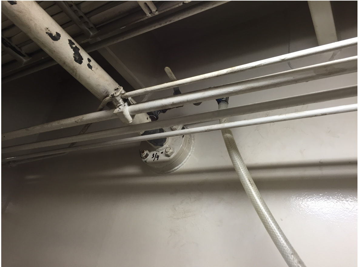
Anolyte dosing point in the water intake pipe
