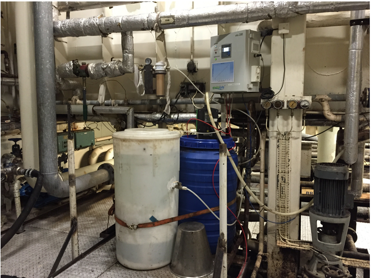
Envirolite ELA-200 anolyte generator on board of M/S SeaWind
