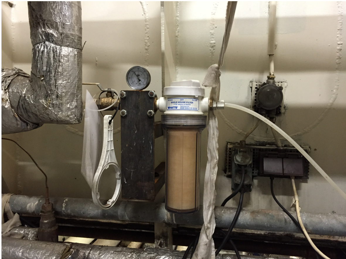
Mains water supply to ELA-200 with filter and pressure controller
