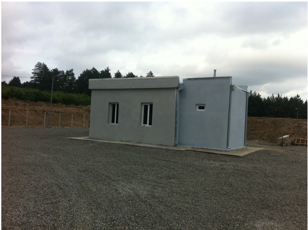
Water purification station
