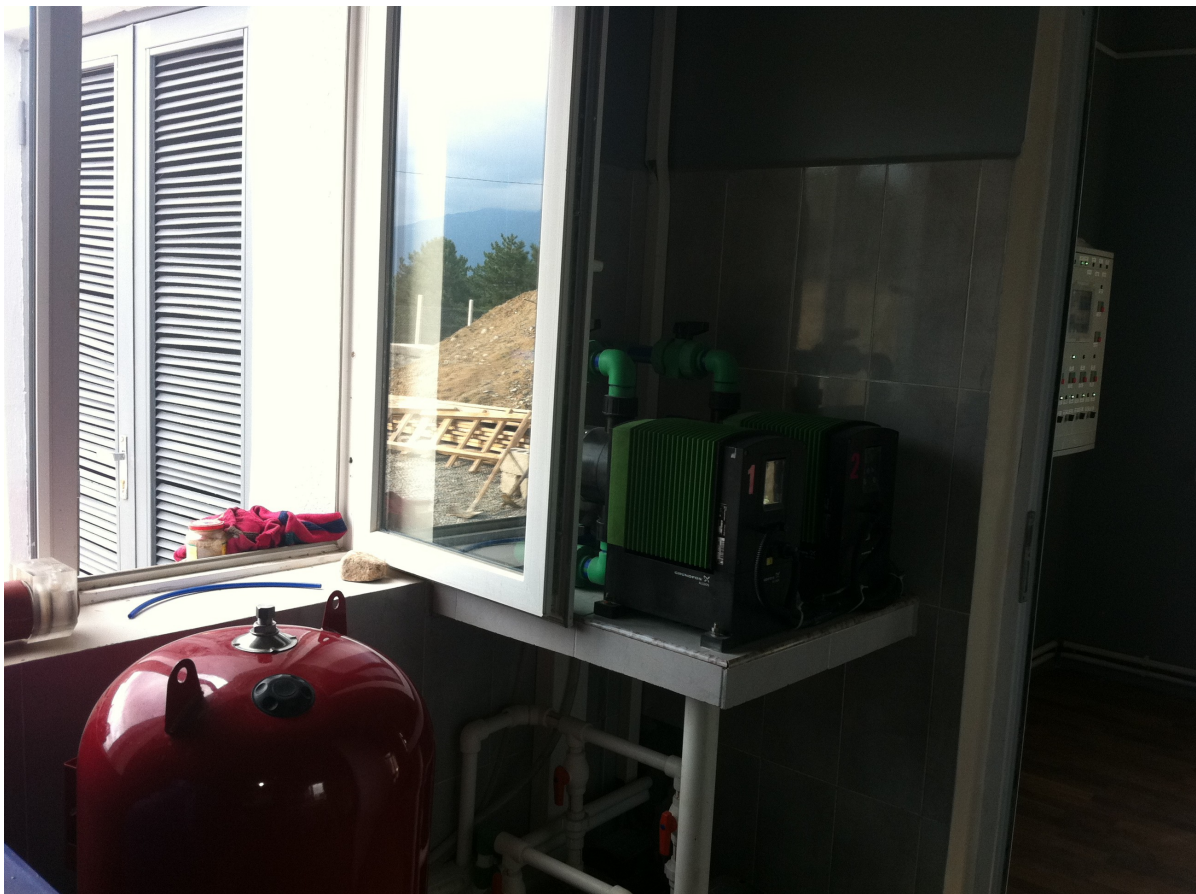
Dosing pumps for analyte
