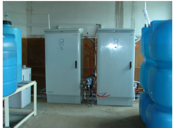
Anolyte tank with level switch (on the right)
