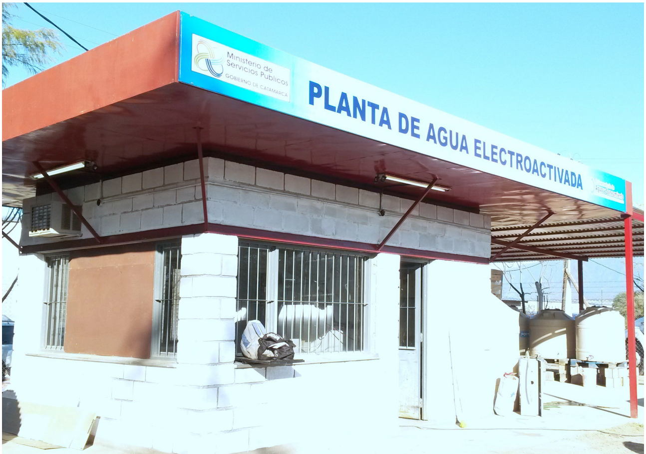
Water purification station
